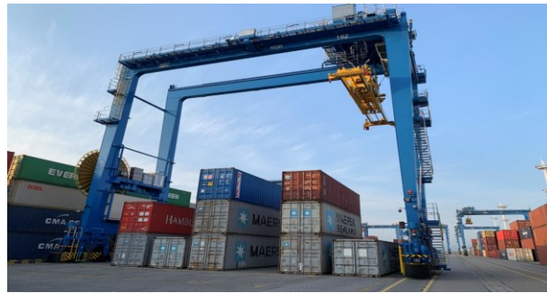
Intelligent gantry crane
